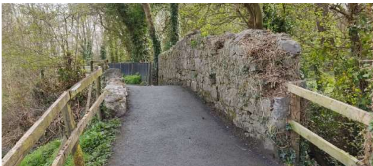
Figure 4-16: View of Bridge 2 from the exiting paved path
