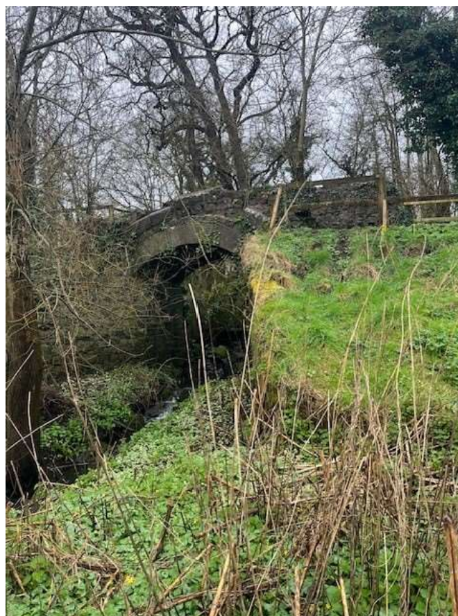
Plate 12-18: Bridge 2 from north side showing vegetation around abutment walls
