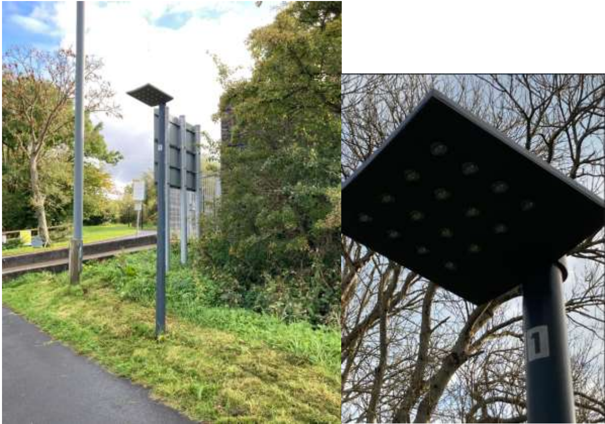
Figure 4-8: Examples of existing Public Lighting Column and Lantern along Limerick Smarter Travel Cycle Route 2
