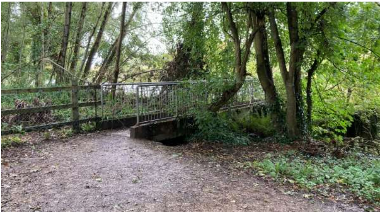
Figure 4-50: Existing concrete bridge at mouth of Plassey mill race looking northeast
