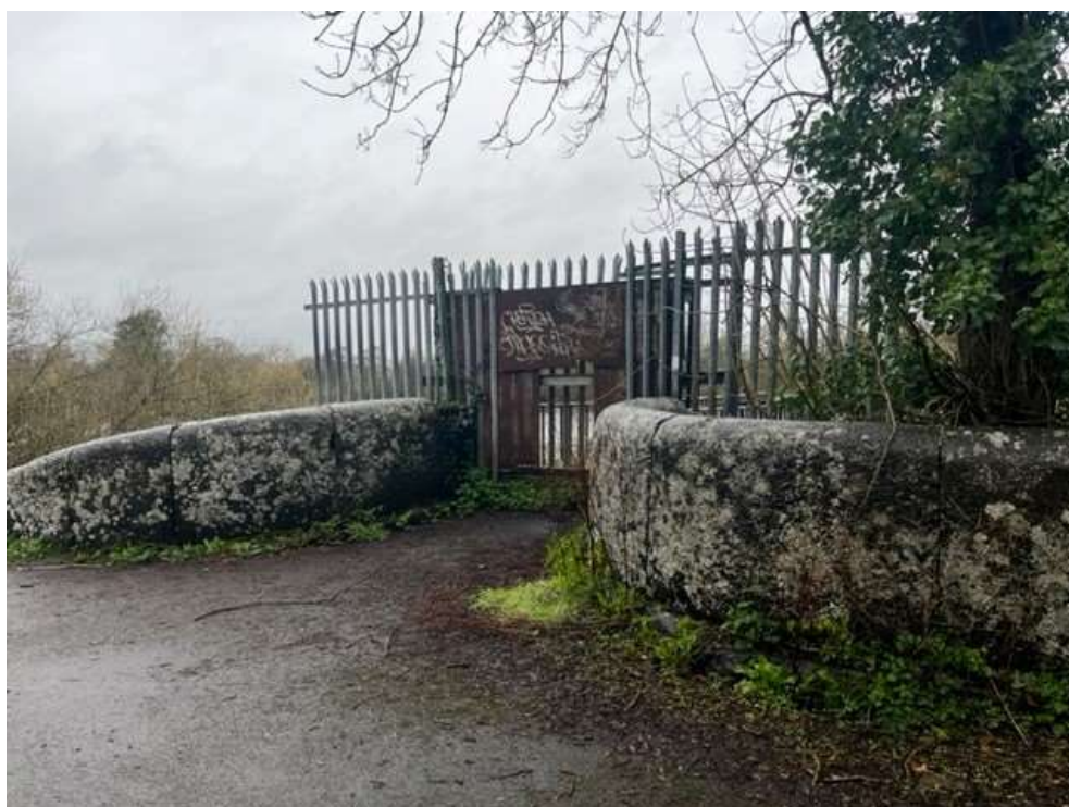
Plate 12-3: Entrance feature onto Plassey Bridge with steel fencing
