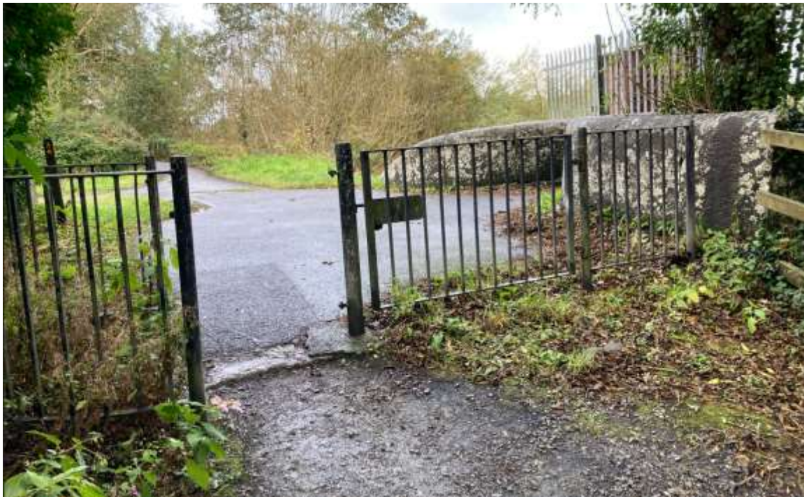
Figure 4-26: Existing gate on path at Plassey Mills (2 of 2)
