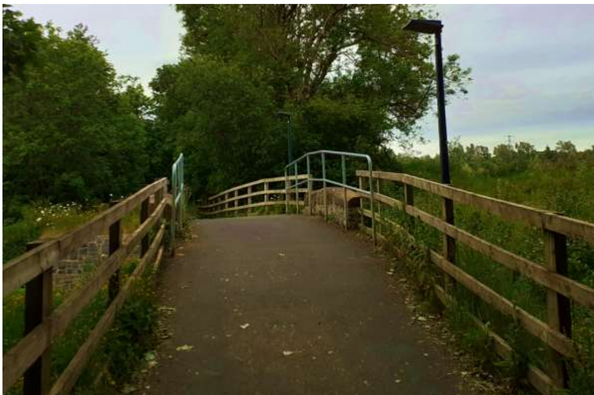
Figure 4-78: Existing bridge at CH400
