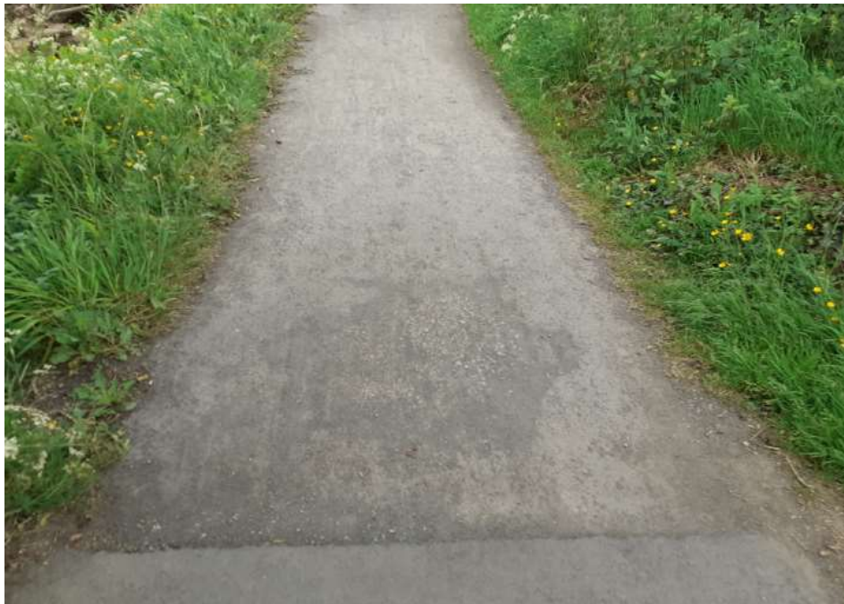
Figure 4-9: Path surface changes from paved to gravel and narrows to approximately 1.5m width
