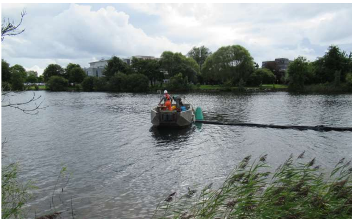
Figure 4-85: Installation of a silt curtain in the River Corrib, Co. Galway
