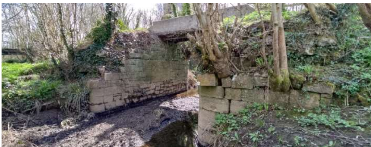
Figure 4-21: Shallow water level in Plassey Mill Race and existing abutments of Bridge 3
