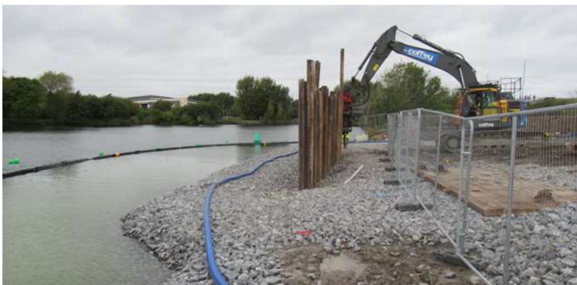
Figure 4-87: Example of sheet piling along the bank of the River Corrib
