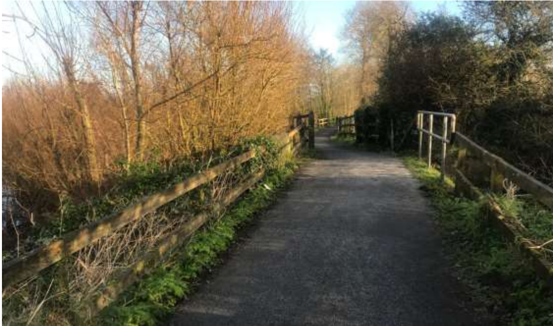
Figure 4-10: Existing Bridge No 1
