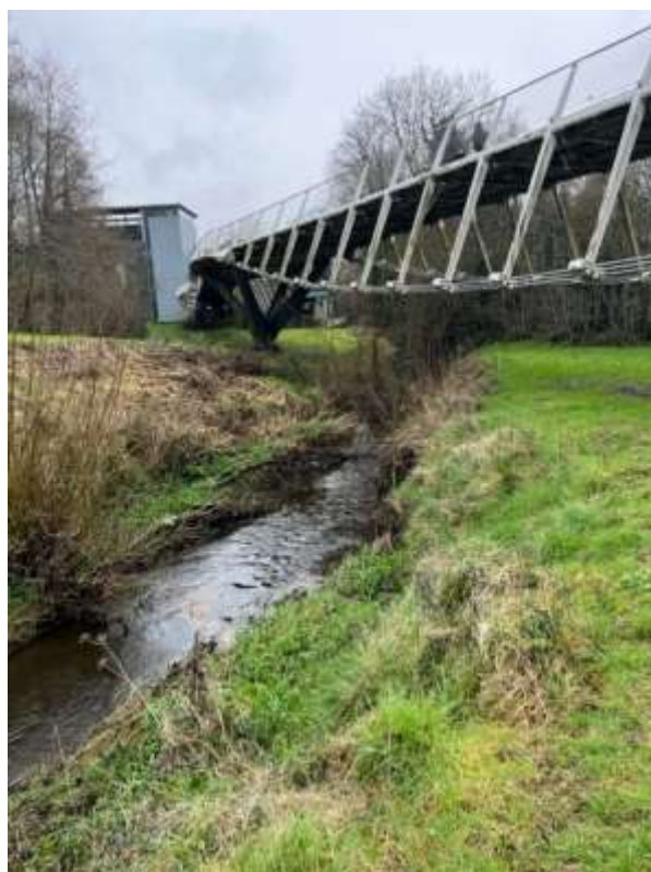
Plate 12-15: Mill Race as it passes beneath footbridge into University of Limerick campus. Very shallow here and no evidence for any masonry walls along this section.
