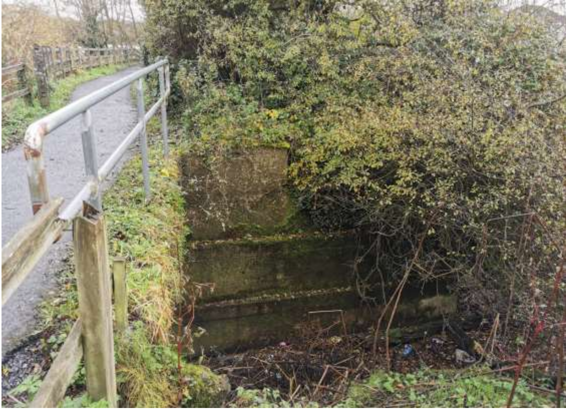
Figure 4-12: Existing abutment wall (proposed to be decommissioned)
