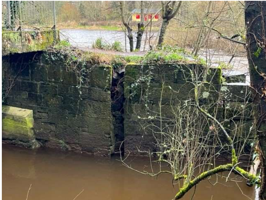
Plate 12-21: Historic masonry linked to mill dam and entrance to mill race from the main river channel
