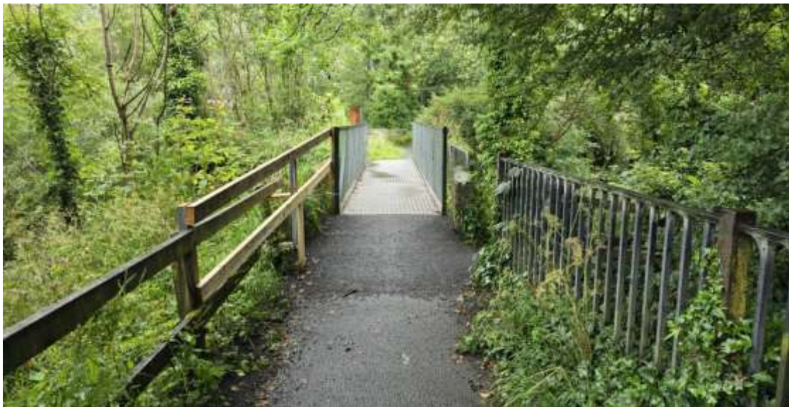
Figure 4-20: Existing temporary bridge across the Plassey mill race where it rejoins the River Shannon
