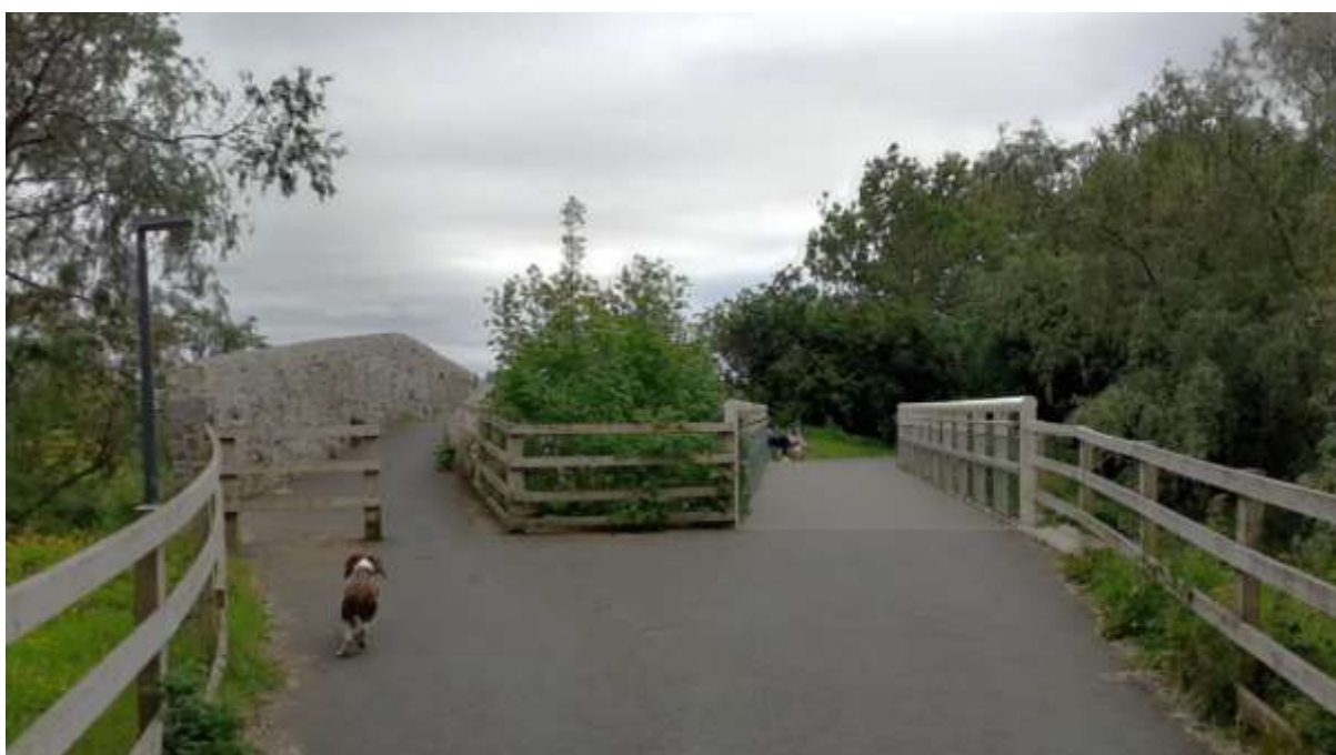
Figure 4-1: Existing Bridge at River Groody
