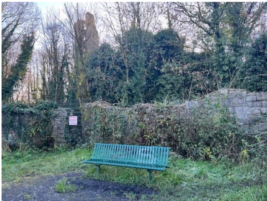
Plate 12-4: Remains of Plassey Mill Building with outbuildings and surrounding wall adjacent to tow path
