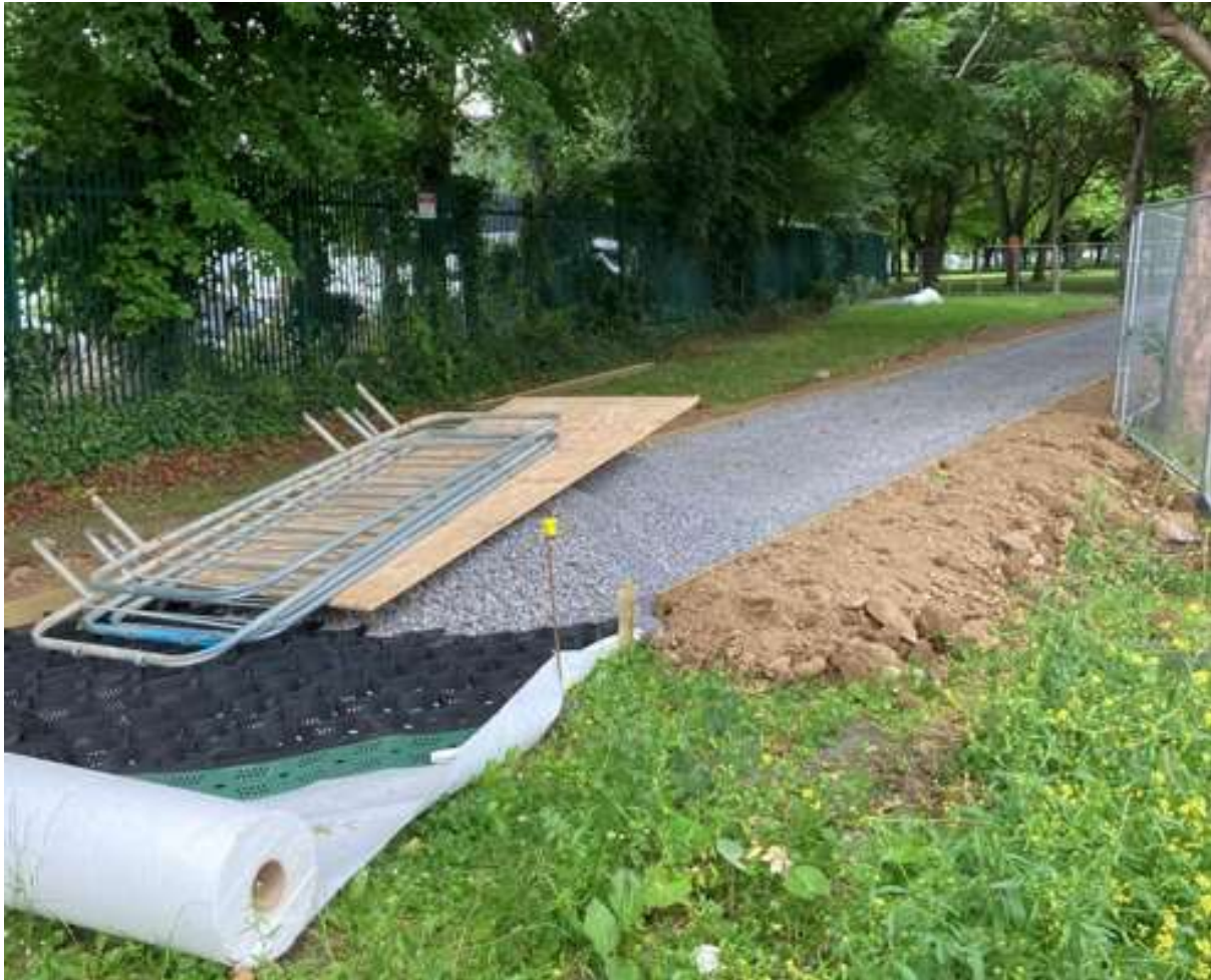
Figure 4-79: Tree root protection system under new tarmac path in Fairview Park, Dublin 3
