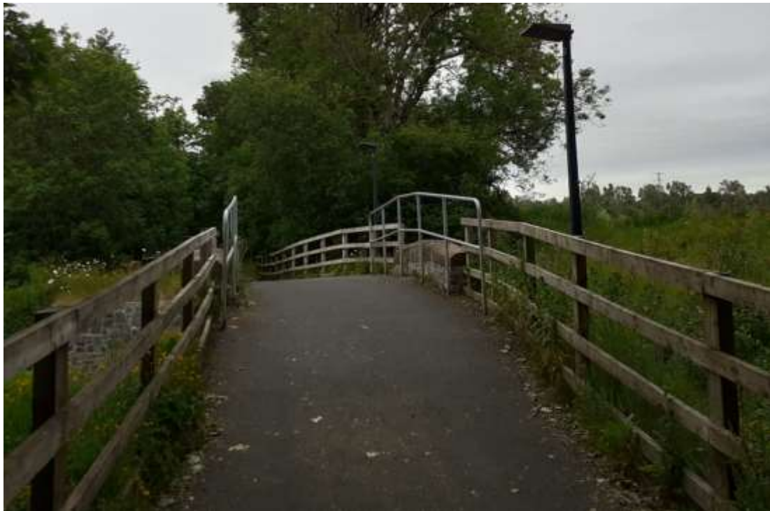
Figure 4-3: Existing bridge at CH400
